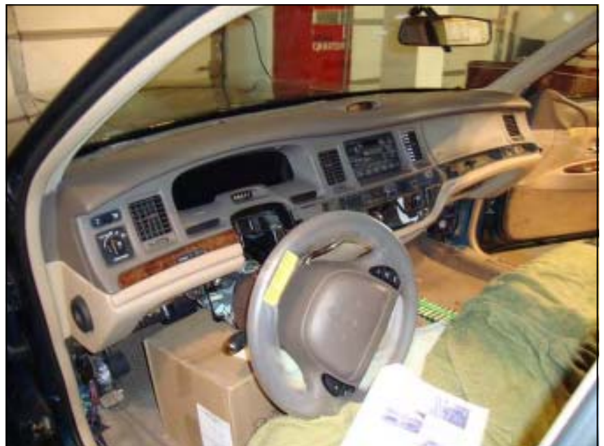
The steering column is lowered and rests on a handy box.
