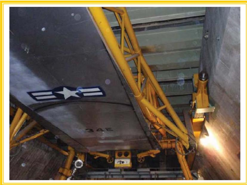
Mock-up of what the missile would have looked like in storage is above. It was held horizontally. If needed, the missile would have been rotated vertically and fueled for launch. This facility and others like it were a one-time use facility. Thankfully it was never used as designed. See vintage photo to the right.
